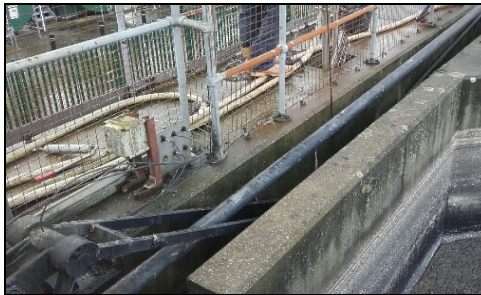
Detritor rake arm and channel
