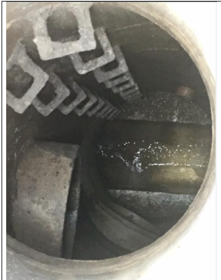
Above - Water was released upstream of a drains chamber in an approved worksite, by a maintenance team unaware of the potential impact to the staff engaged on CCTV survey works. Below – Holding Tank outlet chamber (source of release)
