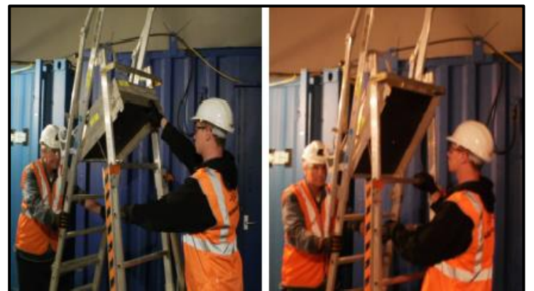
Two operatives dismantling the tower, one either side
