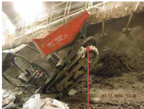
Location of tracked dumper when it came to rest
