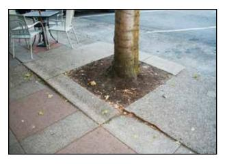
Raised concrete, pavers, and bricks create a trip hazard. Tree roots can raise sidewalks and walkways when a tree is planted too close.
